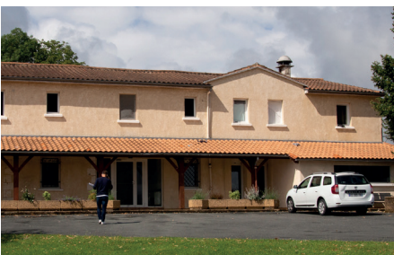
Foyer Mangout – Ribérac (24)
